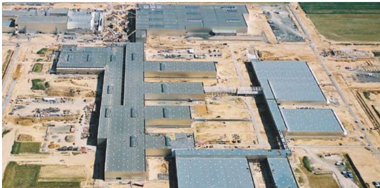
The 85,000 m 2 roof (centre) is safely drained by GM-X steel drainage pipes and JET ® flat roof drains.
